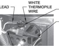
RESETTABLE THERMAL SWITCH **RED THERMOPILE** WIRE
